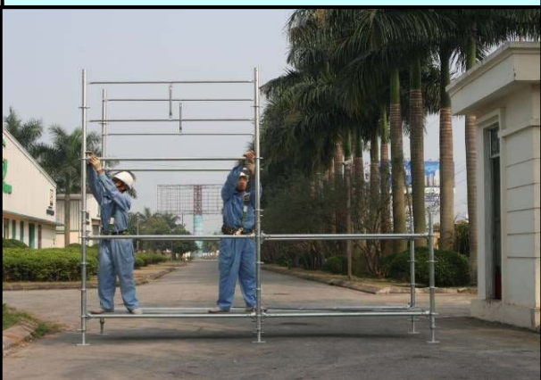
② Fit vertical and set up horizontal
