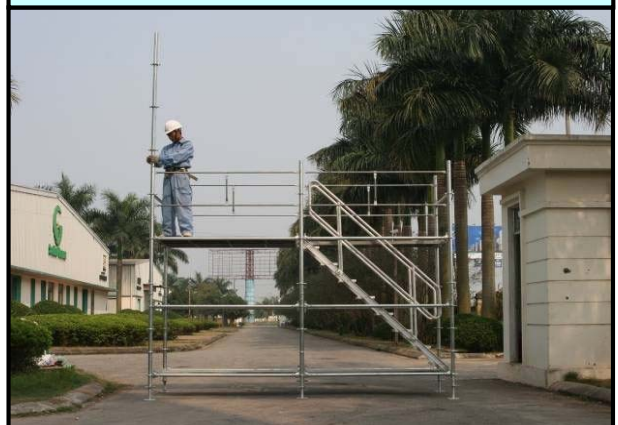
⑥ Set up work stair and finish
