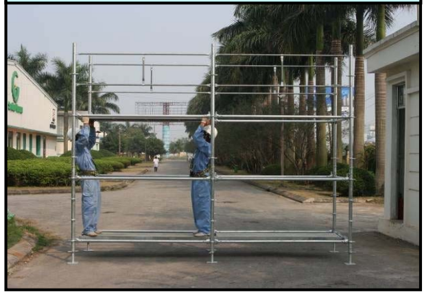
④ Set up scaffold plank
